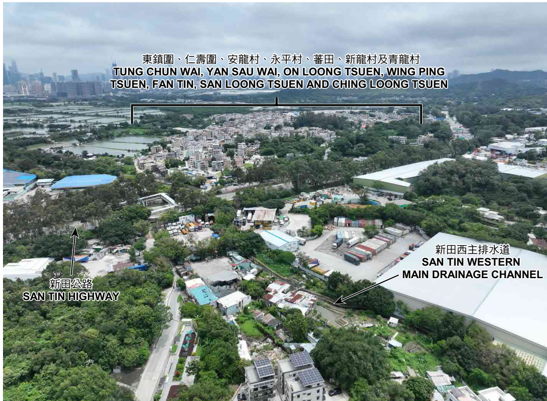
新田公路以南的新田西主排水道 SAN TIN WESTERN MAIN DRAINAGE CHANNEL TO THE SOUTH OF SAN TIN HIGHWAY
