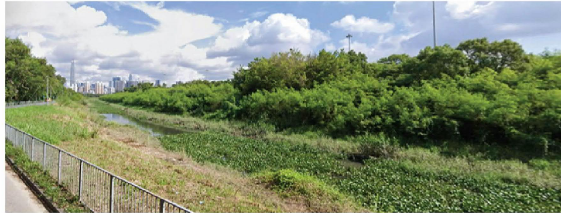
Existing condition- San Tin East Main Drainage Channel
