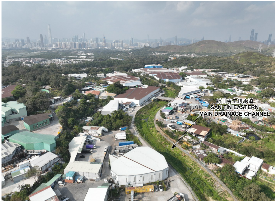
新田東主排水道及鹿尾村一帶 AREA NEAR SAN TIN EASTERN MAIN DRAINAGE CHANNEL AND LUK MEI TSUEN
