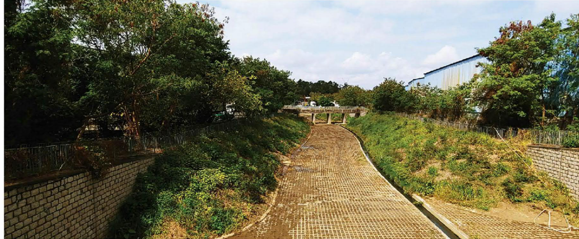
Existing condition- San Tin East Main Drainage Channel
